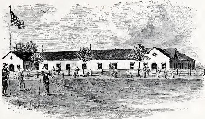
HOSPITAL CAMP, CLEVELAND, 1860-1865
